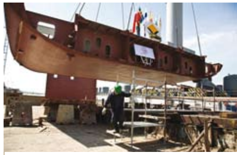
A keel section being laid at Astilleros de Sevilla shipyard in Spain
